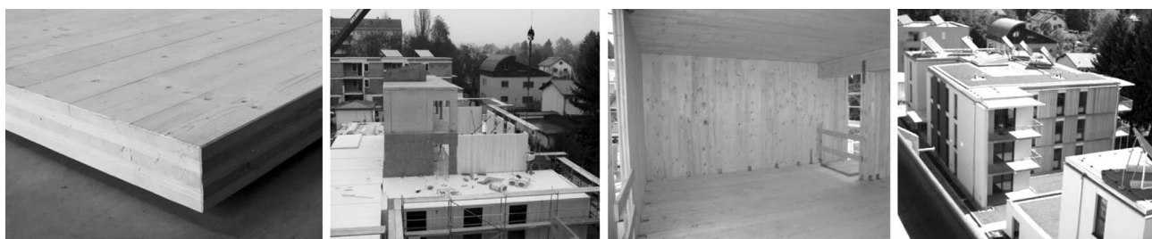
Fig. 1 (Left) five-layer CLT element; (middle to right) impressions from project Wittenbauerstraße/Graz/Austria: two three-storey residential buildings
